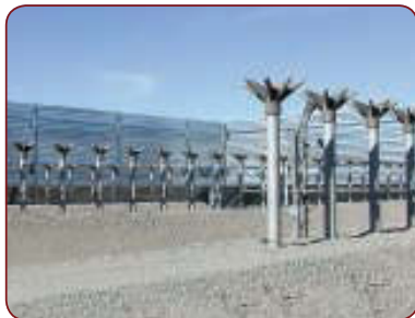
Zeeco multi-point ground flares are often used in olefin facilities
